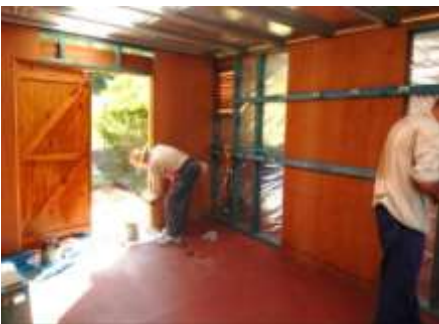
Men at work inside our new Tool Shed in the second car park
